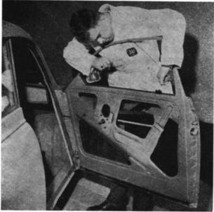
REMOVAL AND INSTALLATION OF DOOR GLASS
